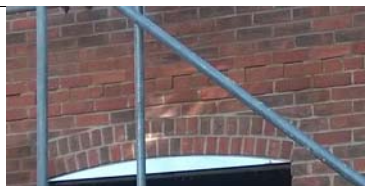
Brick arch over window
